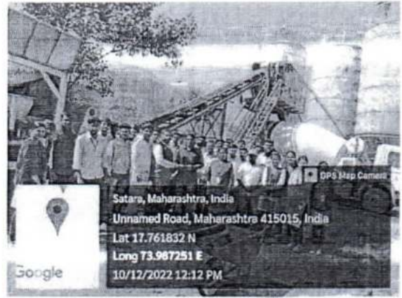
FIG.NO.2 RMC PLANT
