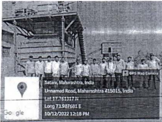
FIG.NO.3 CRUSHING PLANT
