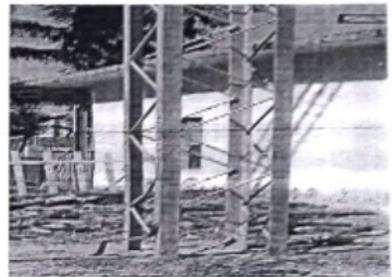
FIG.3 LACING SYSTEM
